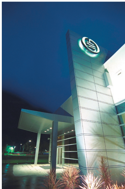
OptiGlobe Telecommunications Rio de Janeiro, Brazil
