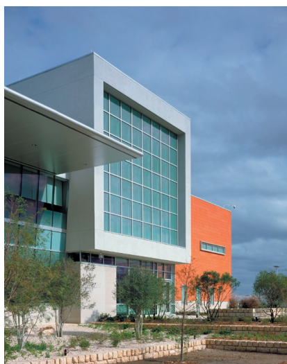
ERCOT I.S.O. Primary Control Center Taylor, Texas
