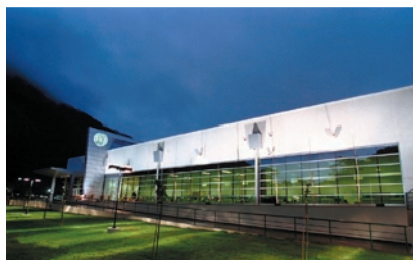
OptiGlobe Telecommunications Data Center Rio de Janeiro, Brazil
