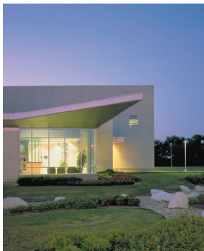
Lower Colorado River Authority System Operations Control Center Austin, Texas
